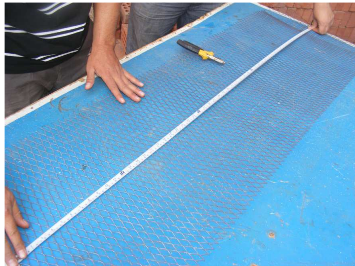
Figure 4: Ferrocement wire mesh
