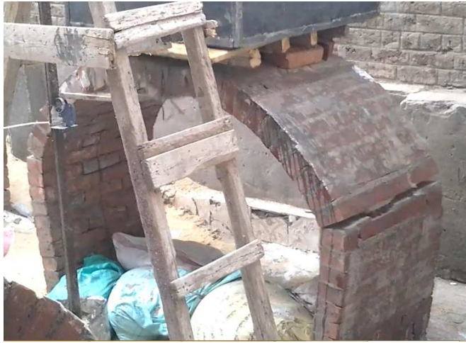
Figure 15: Mode of failure for vaults strengthened by FRP sheets
