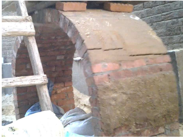
Figure 17: Mode of failure for vaults strengthened by polyester mortar
