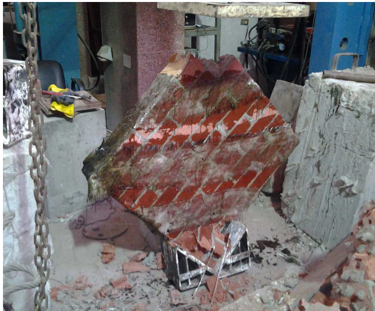
Figure 7: Failure modes for strengthened masonry wallets.
